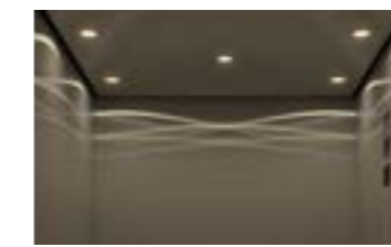
Ceiling: L210S LED downlights (yellow-orange)
